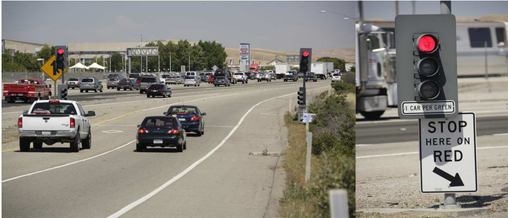
Figure 1.1: Ramp signals on a California freeway. Source: http://www.mtc.ca.gov .
