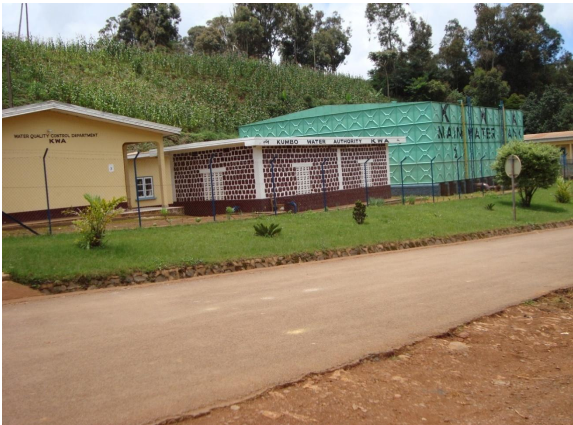
Plate 5 : The Kumbo water purification station and tank (Ngefor G. S., 2011)
