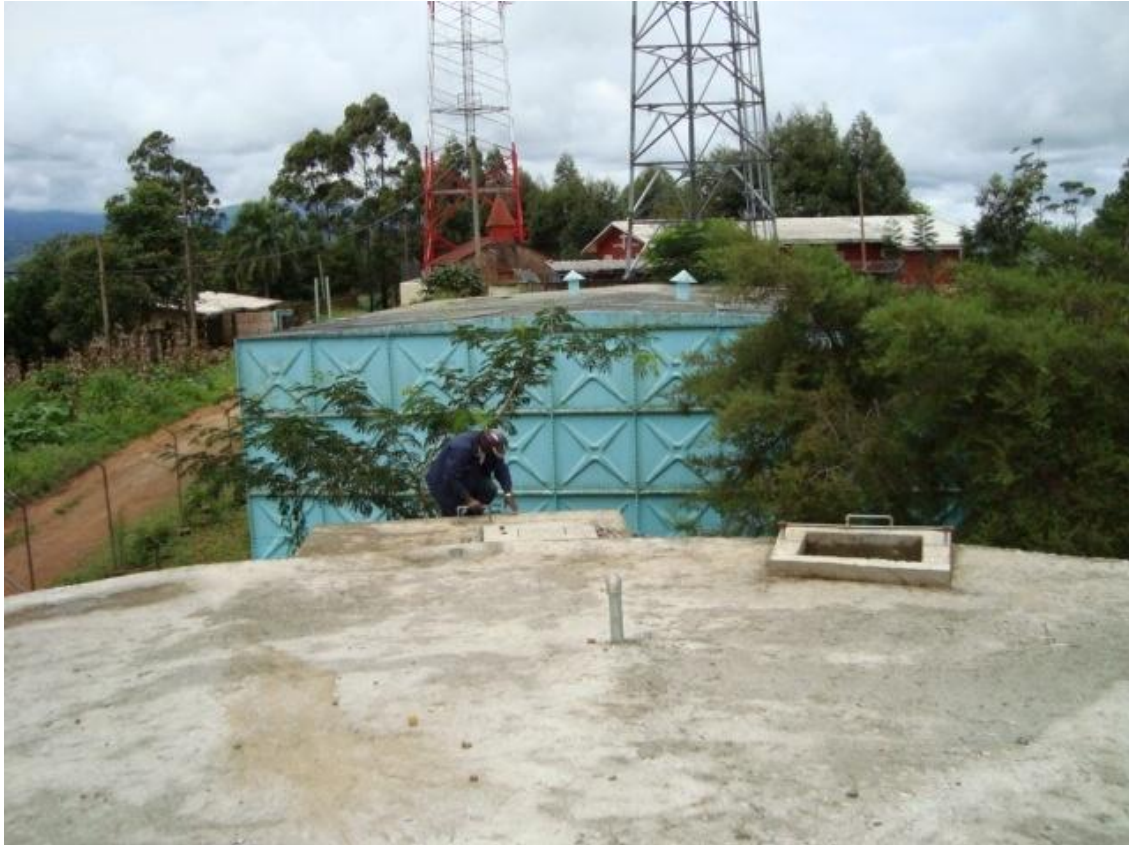
Plate 13: New tank under Construction beside old tank (painted blue)
