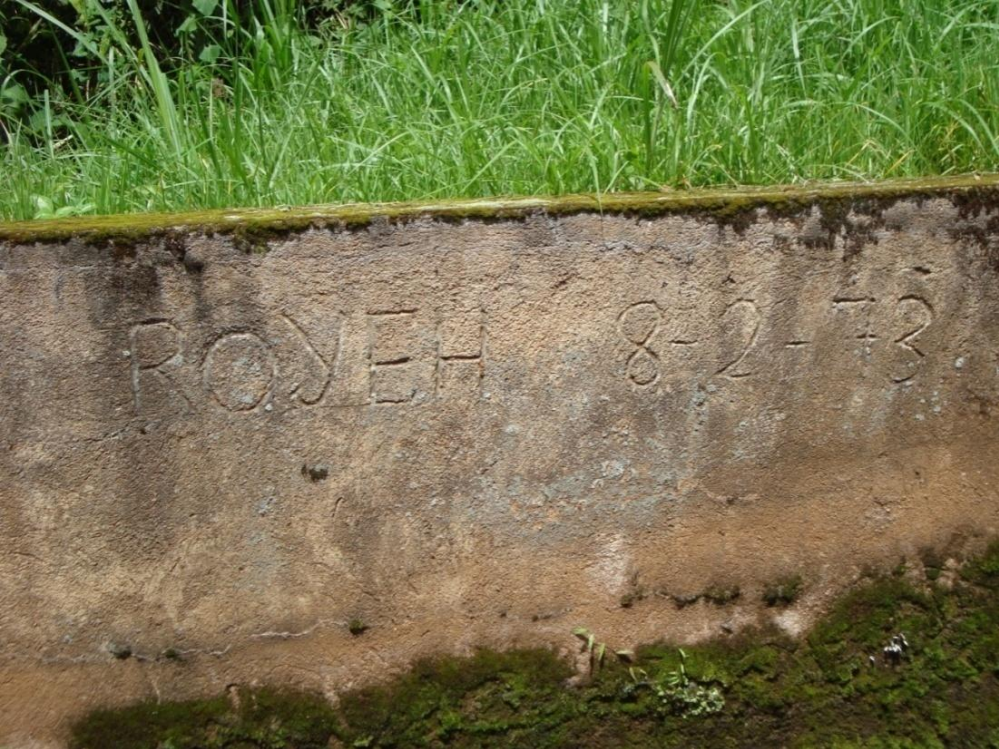
Plate 11 : The Royeh catchment site was constructed a month after the Nonga site to boost the water supply. The catchment sites are managed in Kumbo by the Water Production Department.
