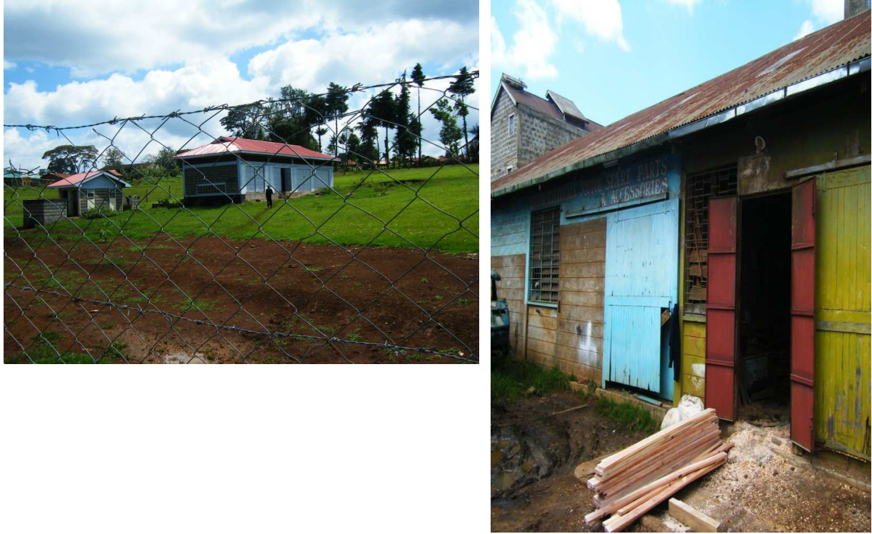
Photo 19: The old and new sheds under construction in Karatina
