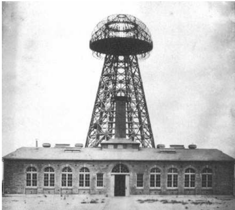
Figure I.1 La Tour Wardenclyffe
