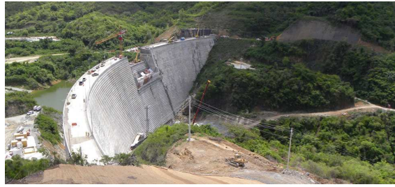
Figure 1.5: Portugues dam, Puerto Rico, USA ( http://www.dragados-usa.com )
