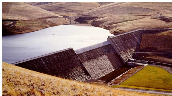
Figure 1.2: Willow Creek RCC Dam, USA ( http://www.nww.usace.army.mil )
