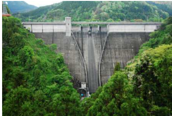
Figure 1.3: Shimajigawa RCD Dam, Japan ( http://damsroom.web.fc2.com )
