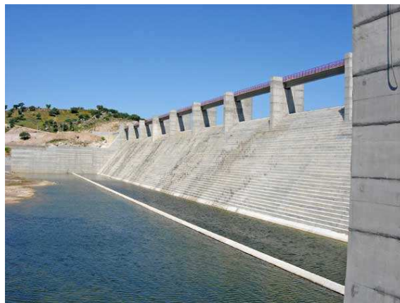
Figure 1.4: Pedrógão dam, Portugal ( http://cnpqb.inag.pt )
