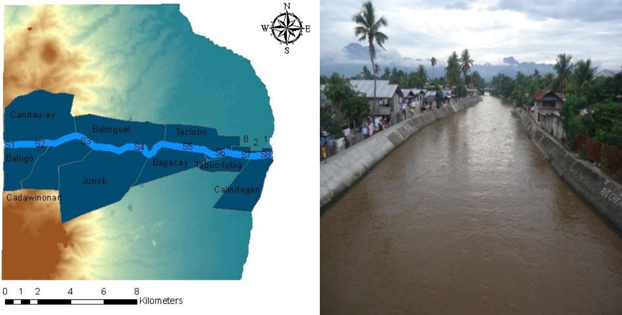
Figure 4-32: Station 8 (S8) Poblacion 1 (Tinago) Bridge
