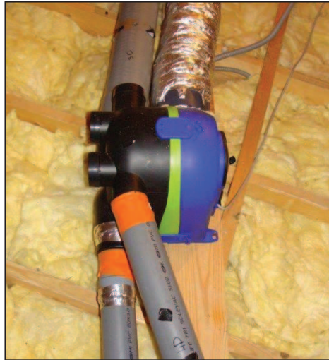
Figure III.6 – Le ventilateur de la VMC HB
