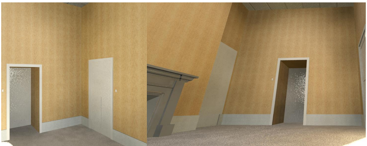
Figure 5.7. Rendering of material components of Gunzo room (existing condition). Wall surface finished by wallpaper and concrete floor finished by vinyl tile
