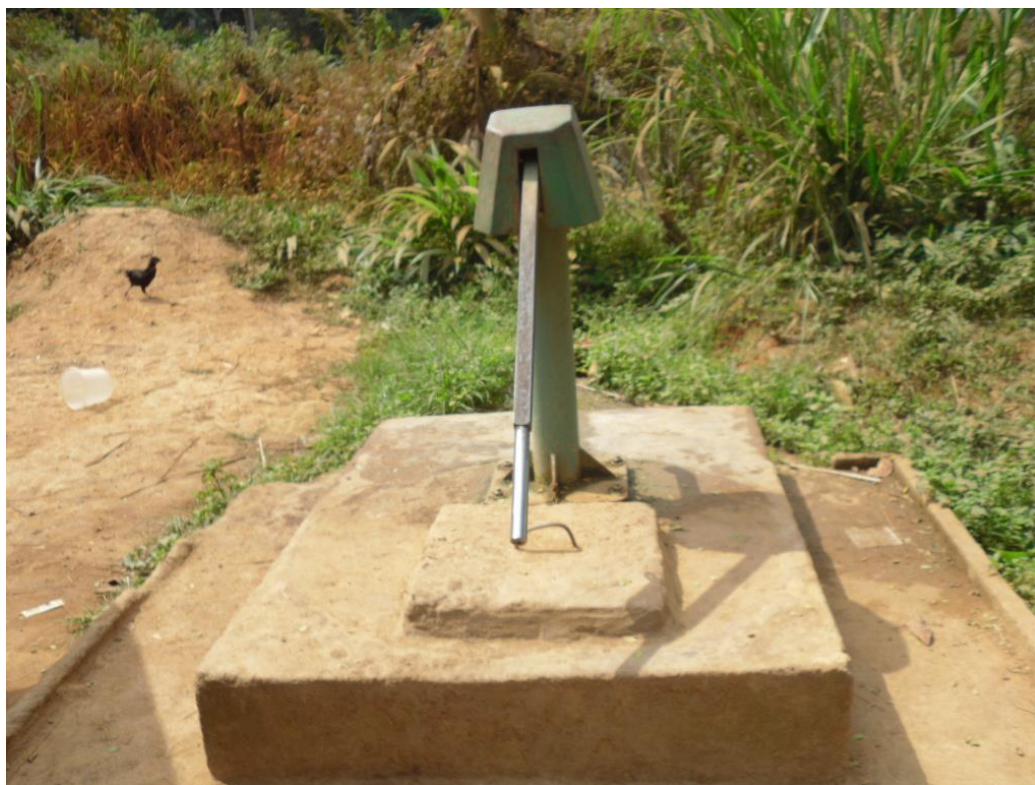
Figure 20 : Forage du village Amvam
