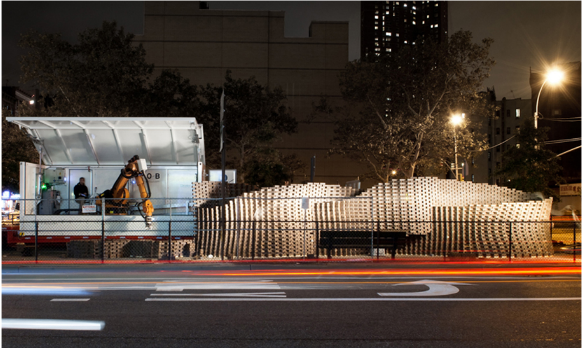
Figure 24. Gramazio & Kohler, Architecture and Digital Fabrication, ETH Zurich, Pike Loop , Manhattan, New York, 2009.
