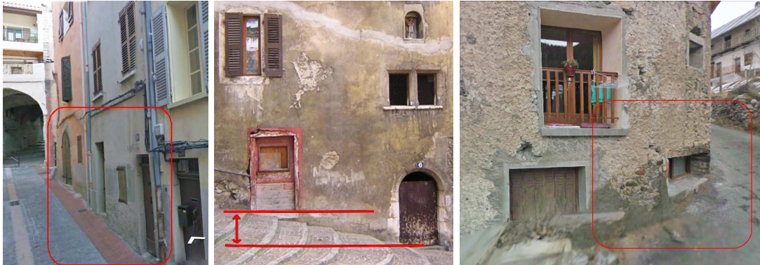
Figure 3.12: Some examples where the architecture of a house has been adapted to the slopes of the underlying terrain.
