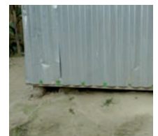
A gap (2.5-5cm) is left between the mud plinth and the fences to protect them from humidity and insects
