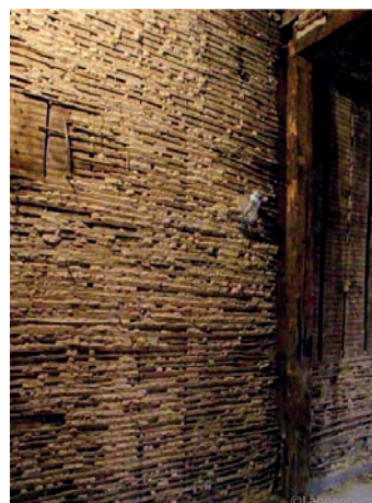
Lattis recouvrant la structure ©Lafont
