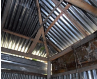
4 slopes roof: in the corner wooden rafters are used to improve wind resistance, others rafters are in bamboo (reduction of the overall cost)
