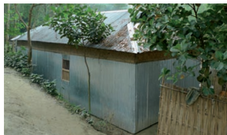
Due to the limited length of the CGI sheets, jute sticks or bamboo woven fences are placed on the top of the wall (40cm) to get a greater height and to improve ventilation of rooms
