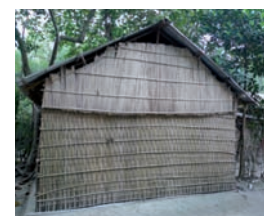
A gap (2.5-5cm) is left between the mud plinth and the fences to protect them from humidity and insects
