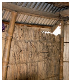
A gap (2.5-5cm) is left between the mud plinth and the fences to protect them from humidity and insects
