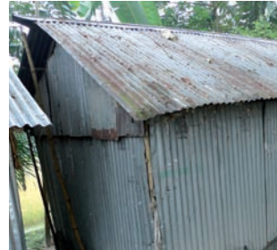
4 slopes roof: in the corner wooden rafters are used to improve wind resistance, others rafters are in bamboo (reduction of the overall cost)
