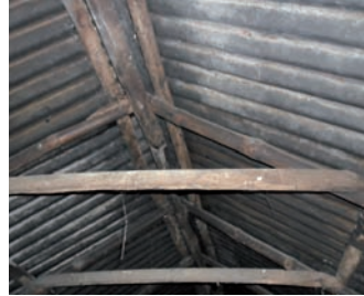
4 slopes roof: in the corner wooden rafters are used to improve wind resistance, others rafters are in bamboo (reduction of the overall cost)
