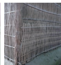
A gap (2.5-5cm) is left between the mud plinth and the fences to protect them from humidity and insects
