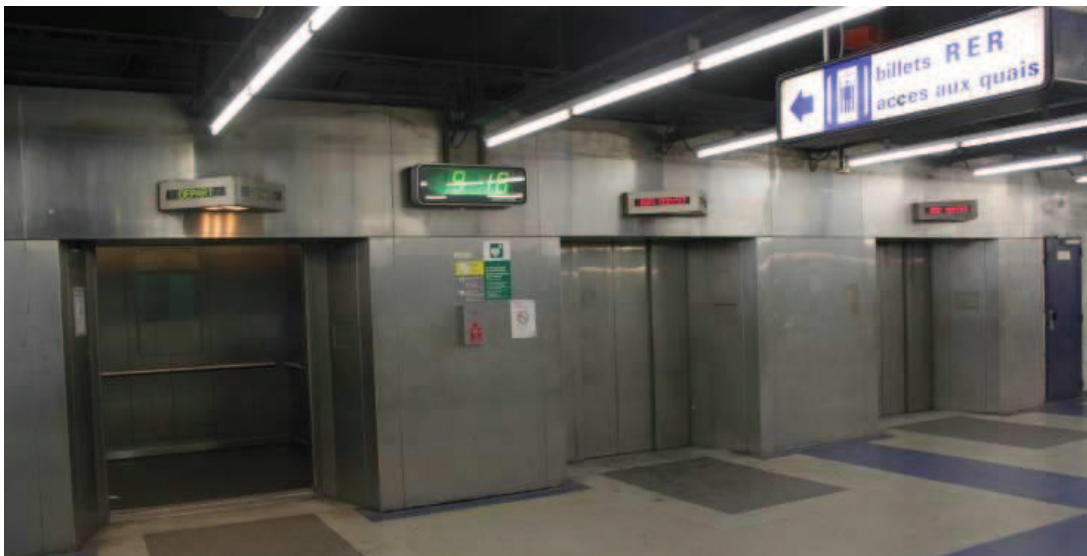
Figure 15: Elevators for primary use in Paris, Auber station (source: author)
