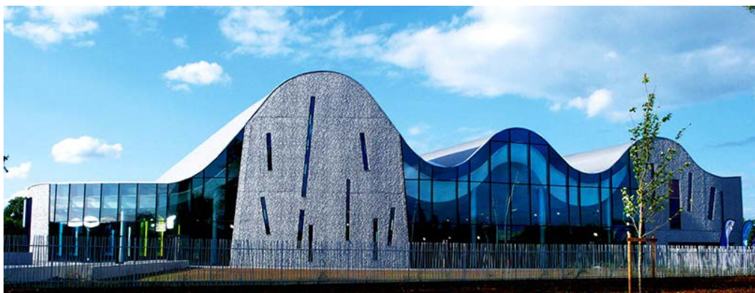
Figure 3.1: What is the differential equation describing the roof of Aquarena swimming pool in Arras?
