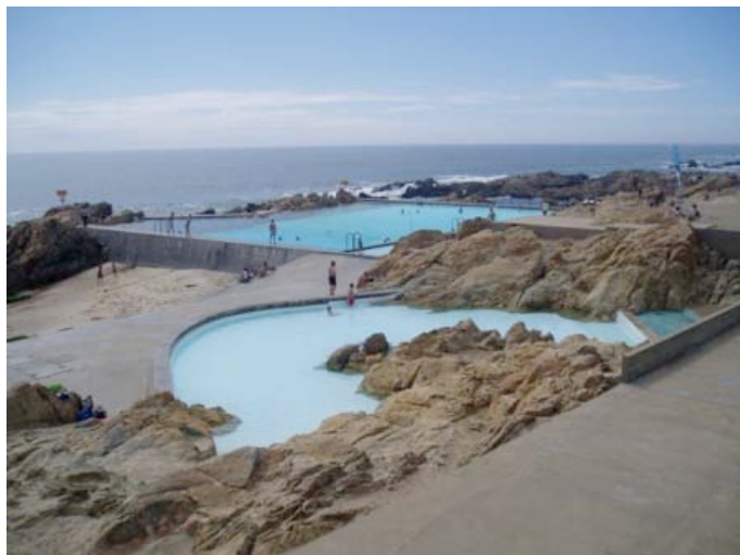
Figure 7, Siza A. Source, Swimming pool. http://alvarosizavieira.com/1966-leca-swimming-pools
