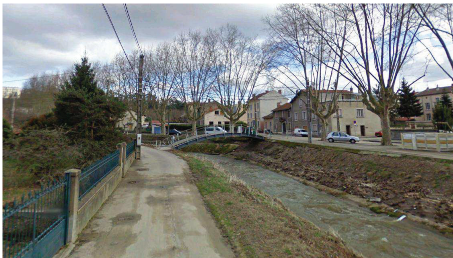
Figure 6.16 : Small bridge at stage gauge L_2 location photographed after the 2009 flood (Source: Google Map)
