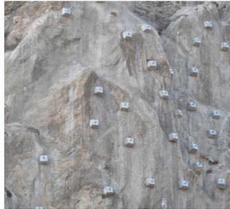
FIGURE 2.3 – Les ancrages scellés [DESPLOM]
