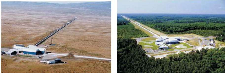
Fig. 29. – (Colour online) Aerial photographs of the LIGO observatories at Hanford, Washington (left) and Livingston, Louisiana (right). The laser sources and optics are contained in the blue and white buildings. From these buildings, evacuated beam tubes extend at right angles for 4 km in each direction, which are covered by concrete enclosures. Photos taken from ref. [97], courtesy of the LIGO scientific collaboration.
