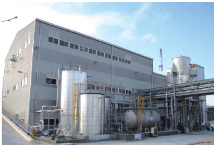
Figure I-33. First commercial plant (1000 tons per year) for the continuous supercritical hydrothermal synthesis of \text{LiFePO}_4 ; plant was constructed by Hanwha Chemical [207] Copyright © 2011, Royal Society of Chemistry.
