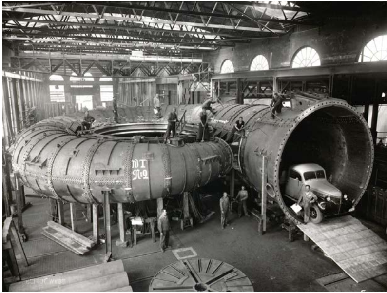
Figure 1.5: Spiral casing produced by the company Escher-Wyss (Zurich) in 1938 for the Sungari powerplant in Manchuria.
