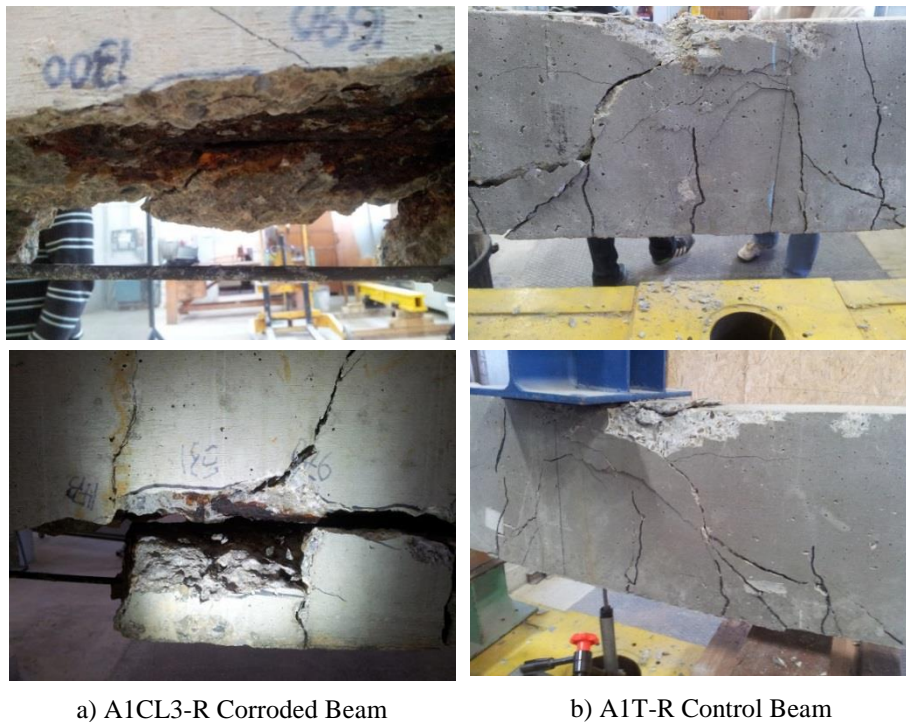
Figure 2 - 7 Modes of failure and damages of two full span beams A1CL3-R and A1T-R
