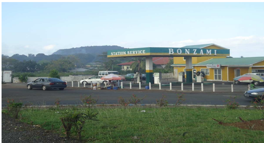
Ph. 64. La seconde station de carburant de Malouzine
