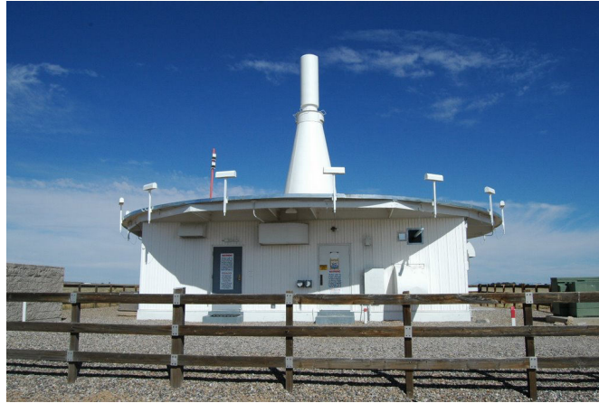
FIGURE B.1: VHF Omnidirectional Range ground station 4
