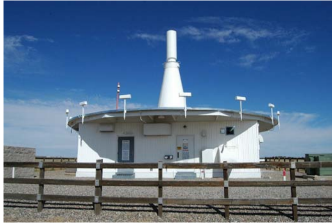
FIGURE B.1: VHF Omnidirectional Range ground station 4
