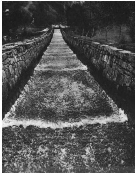
Figure 5.9: Roll waves flow down an inclined channel by Grönnbach, Merlingen (Suisse) in [12].
