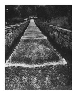
Figure 5.9: Roll waves flow down an inclined channel by Grünnbach, Merlingen (Suisse) in [12].
