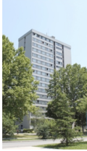
Figure 6.3: Perspective view of Arpej II tower in Grenoble (France).
