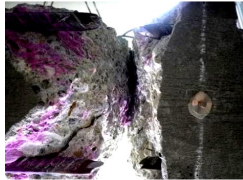
(b) non-corroded beam
