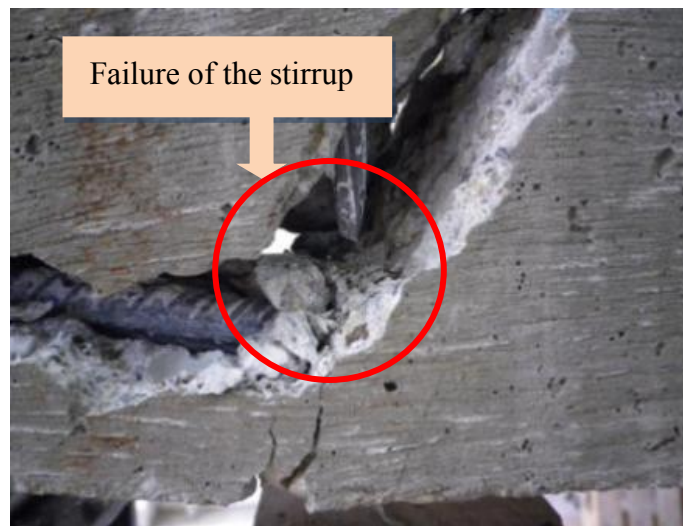
Figure 7-5 Failure point of the stirrup of the non-corroded beam (B2T2-2)
