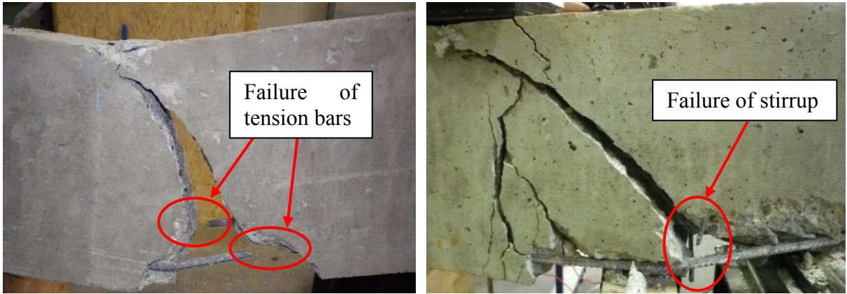
(a) Failure of non-corroded beam B2T3-1 (b) Failure of non-corroded beam B2T3-2
