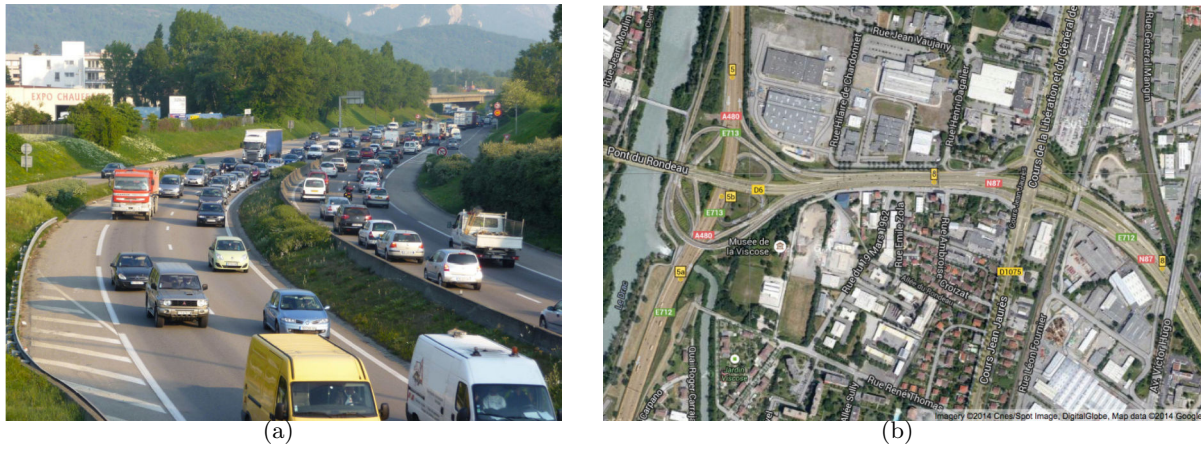
Figure 1.4: The south ring of Grenoble. (a) View of a stretch of the south ring, direction north-east towards Meylan (image courtesy: DIR-CE); (b) Aerial view of the interchange “Rondeau” at the west end of the south ring (left, center): this site experiences heavy traffic congestion during the morning and afternoon rush hours, which may propagate upstream for several kilometers (source: Google Maps/Satellite).
