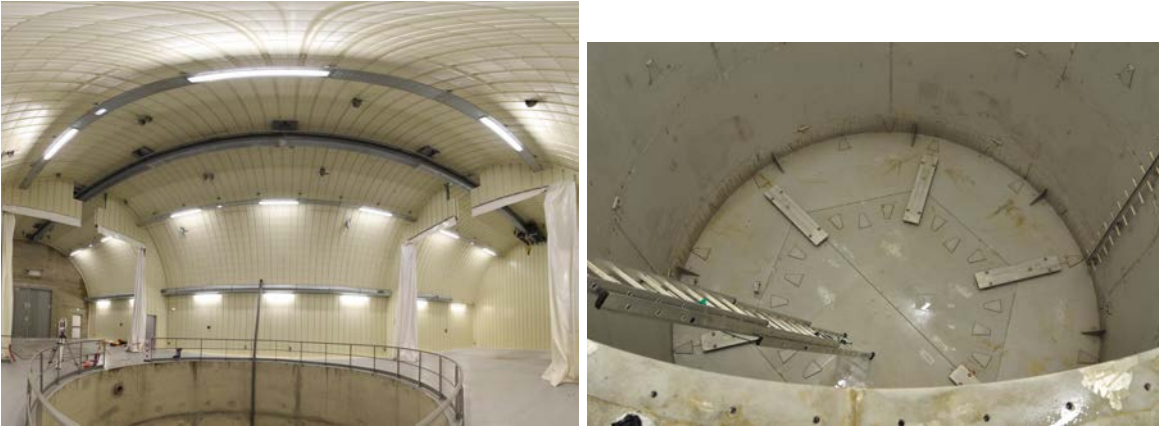
Figure 6.3: Left: Near laboratory upon delivery. Right: Inner Veto supports installed in the pit.
