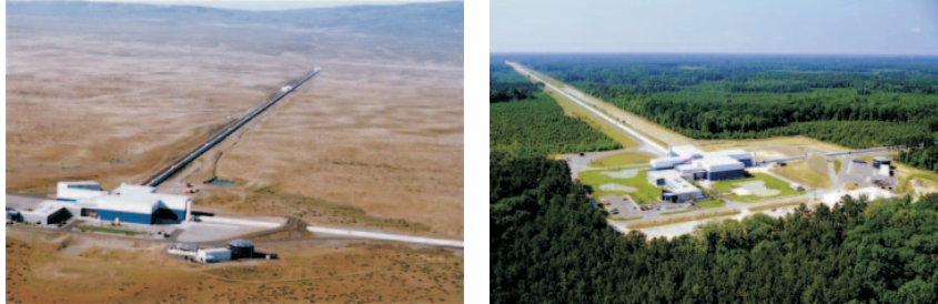
Fig. 27. – (Colour online) Aerial photographs of the LIGO observatories at Hanford, Washington (left) and Livingston, Louisiana (right). The lasers and optics are contained in the white and blue buildings. From the large corner building, evacuated beam tubes extend at right angles for 4 km in each direction which are covered by the arched, concrete enclosures. The full length of only one of the arms is shown in each image. Photos courtesy of the LIGO scientific collaboration.
