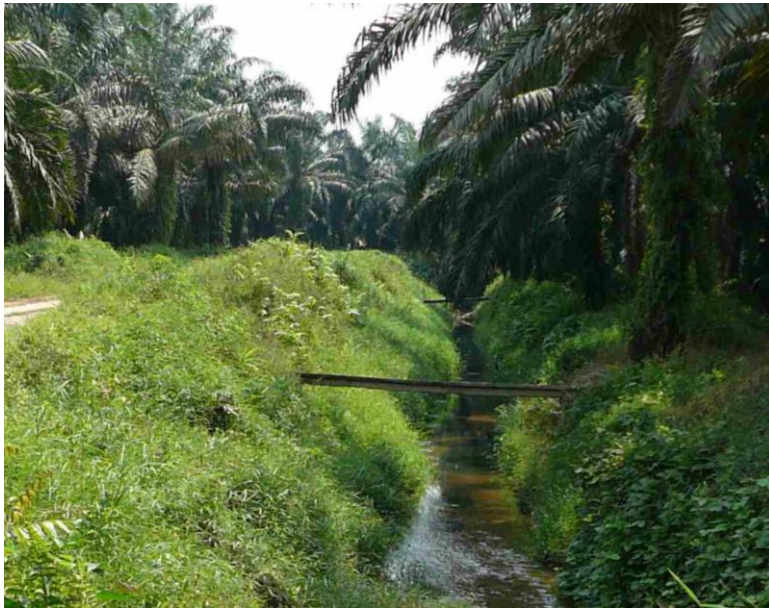
Drainage ditch with narrow cement bridge (Riau_2 plantation)
