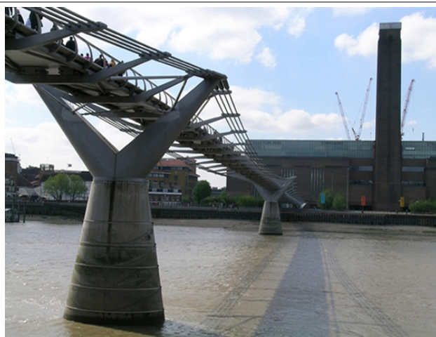
Image du Millennium foot bridge, source : http://resoundings.org/Pages/Harmonic_Bridge1.htm
