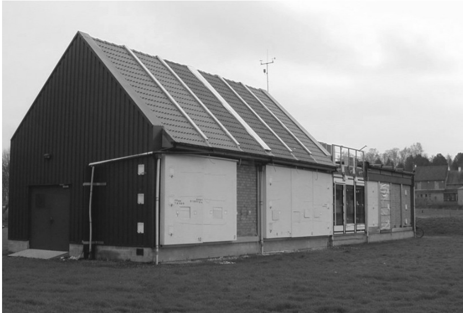
FIGURE 1.6 – VLIET Building (Blocken and Carmeliet, 2005)
