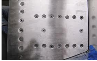
Figure 5.3: Fastened rivet holes.
