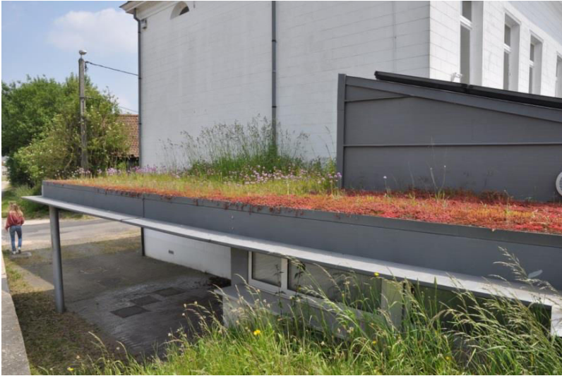
Fig. 1.3 An EGR installed on a carport in Flanders, Belgium. Micro variation in environmental conditions clearly influences vegetation composition [Picture: Frederik Lerouge; Division of Forest, Nature and Landscape; June 2013].
