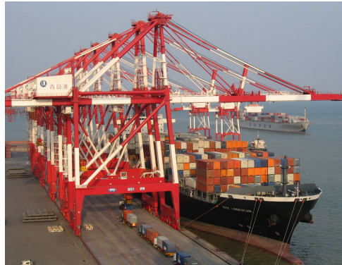
FIGURE 8 – Grue de quai
