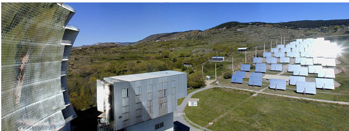
Figure 5.3: Photograph of Odeillo's 1 MW solar furnace.
