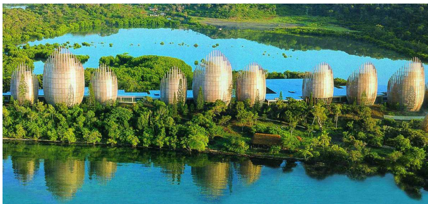
Figure 1.13 – Centre Jean-Marie Tjibaou à Nouméa
