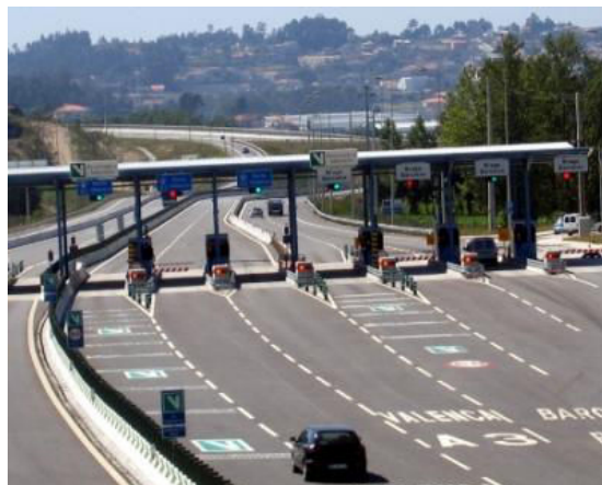
Fig. II-2. Stop&Go toll collection configuration.
