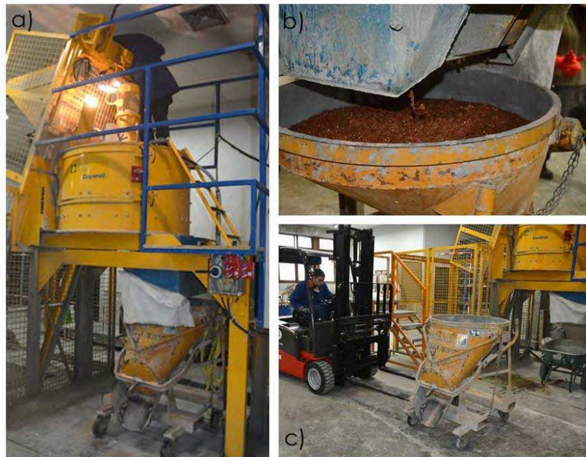
Figure 21. a) 200L mixer and the concrete bucket; b) Filling of the concrete bucket with the geopolymer concrete c) Forklift lifting the full bucket.
