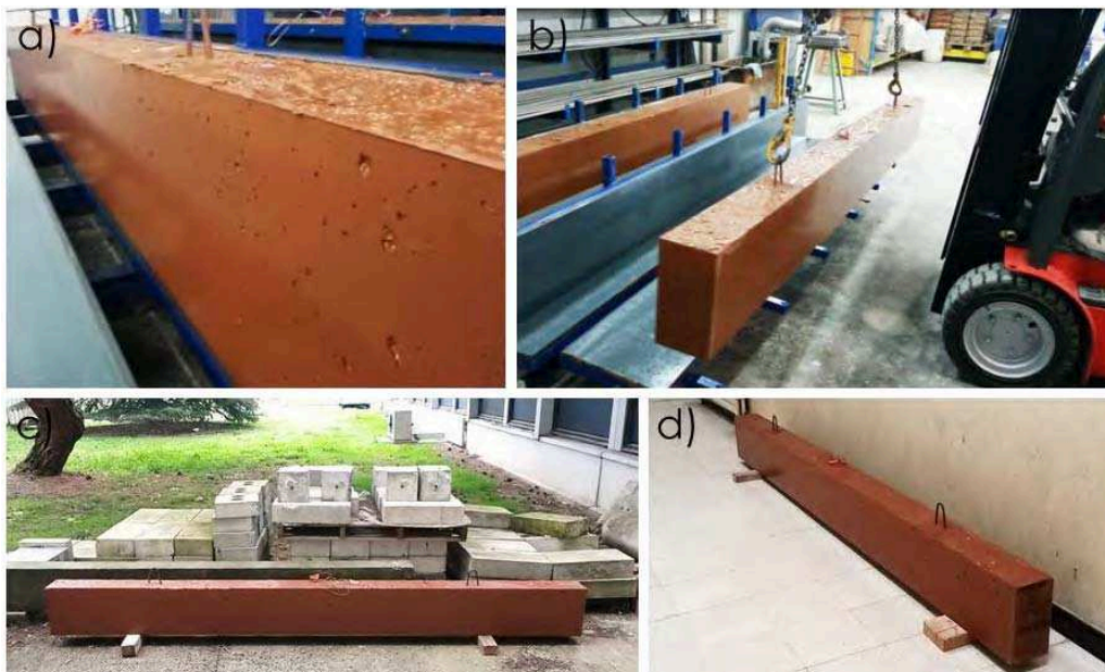
Figure 23. a) side of B1 showing the air bubbles trapped in the fresh concrete b) beam B1 removed from its mould using a forklift; c) B1 stored outdoors and d) B2 stored indoors.
