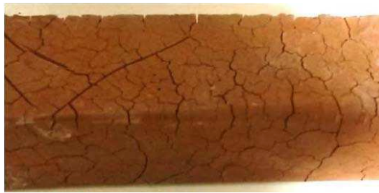
Figure 24. Marked surface cracking on geopolymer mortar due to drying shrinkage
