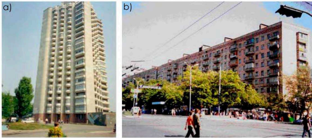
Figure 2. (a) The first residential building made of alkali-activated cement concrete without any OPC, Lipetsk, USSR, 1987–1989 (b) One of two 9-storey residential buildings, Mariupol, Ukraine, 1960 (Palomo et al, 2014).
