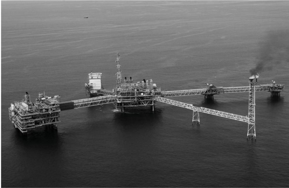
**Figure 1.4:** Aerial view of the Total offshore platform located in Amenem (Niger's Delta). The natural gas obtained as a byproduct of the oil extraction is burnt (right side of the picture). (Pius Utomi Ekpei/AFP/Getty Images, [www.theatlantic.com](http://www.theatlantic.com))
