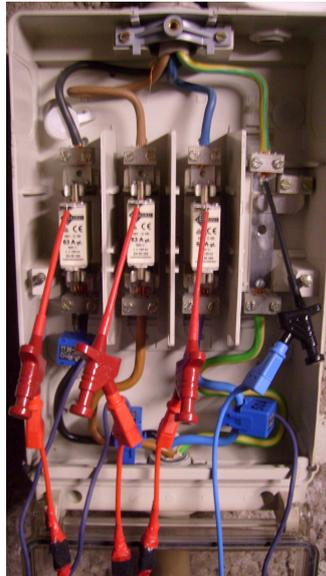
Figure A.2 – Measurement in a residential building. The sensors are plugged directly to the household entry point. The voltage and current of three phases were measured.
