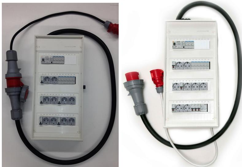
(a) Switching and detection box 1, consist of 10 standard outlets.
