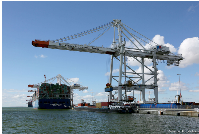
Figure I.11 – Grue de quai
