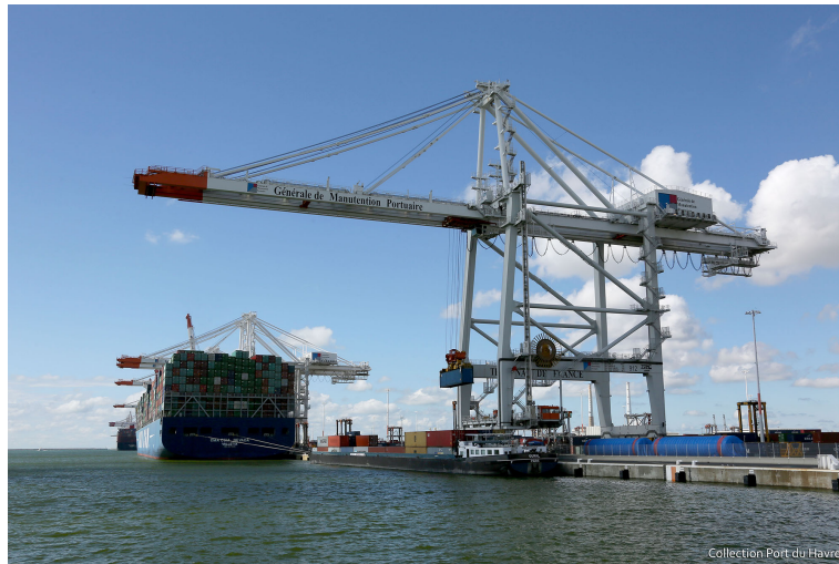
Figure I.11 – Grue de quai
