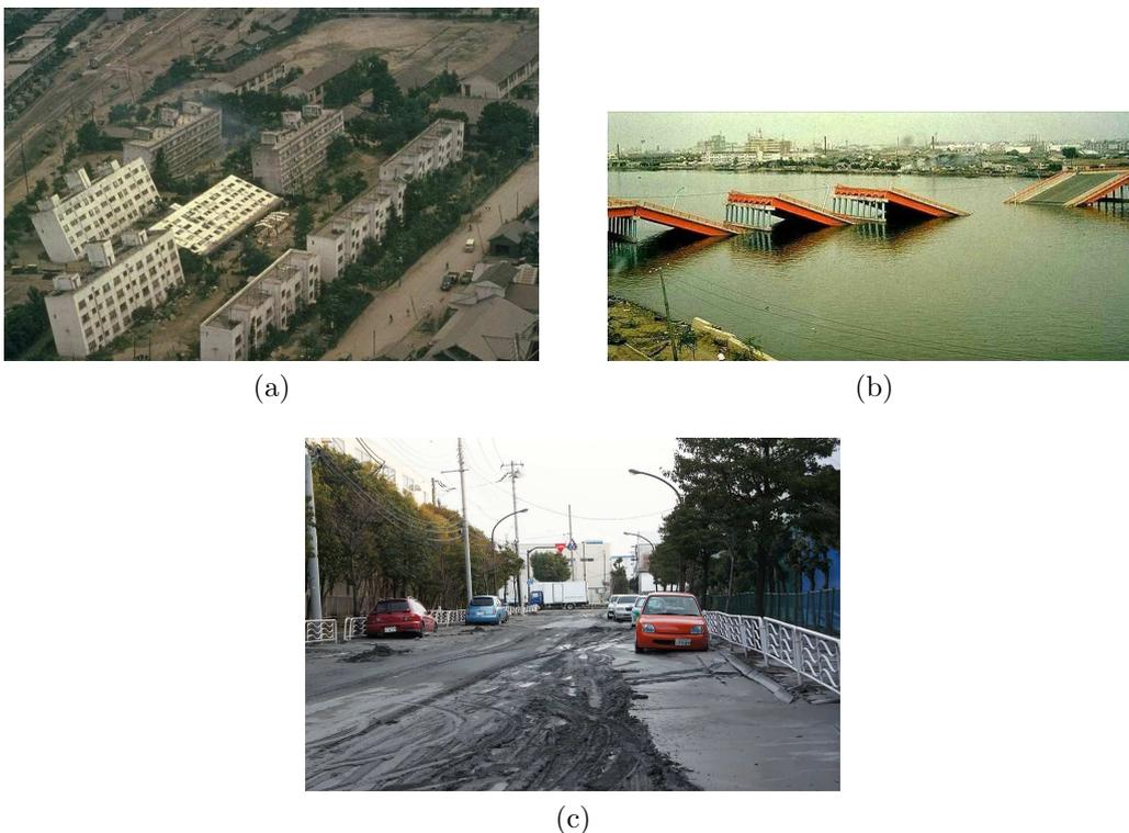
Figure 2.1: Liquefaction-induced damages: a) Ground failure caused buildings to suffer bearing capacity failures and tilt severely after Niigata earthquake in 1964 ( $M_w=7.5$ ), b) Lateral spreading caused the foundations of the bridge to move laterally and collapse after Niigata earthquake in 1964 ( $M_w=7.5$ ), c) Ground failure caused damages to roads in Koto, Tokyo after the 2011 Tohoku earthquake in Japan ( $M_w=9.0$ ).
