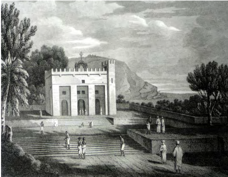
Fig. 3.11 (a) Stela 7 with the relief of “house” (top, left); two stone thrones at the church enclosure (top, center) and throne 9 (top, right); base plate of stela 4 (lower, left); and base of column (lower, right) (adapted from Salt, 1814); (b) view of Aksum Maryam Tsion from west as illustrated by Salt in 1805. Behind the church at the background stands the hill of May Koho while the standing stela of the south-east stela field can be seen at the right lower edge of the hill (adapted from Valentia, 1809).
