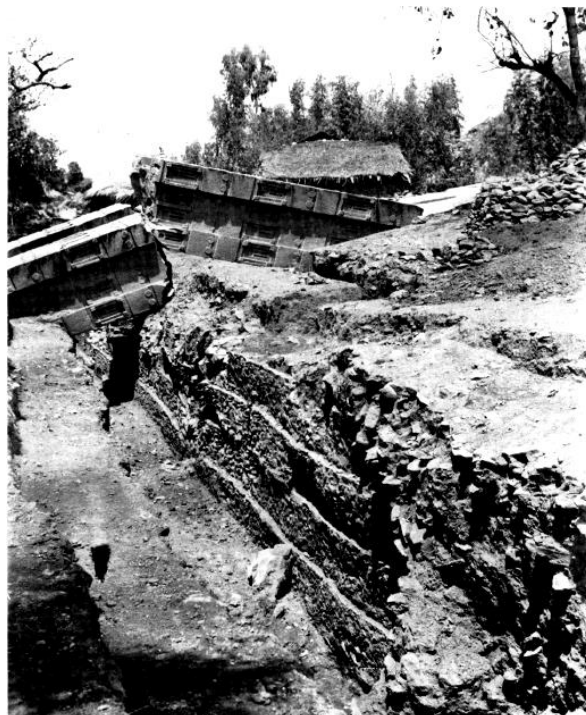
Fig. 4.7 The excavation of wall M1, viewed from east (adapted from Leclant, 1959).
