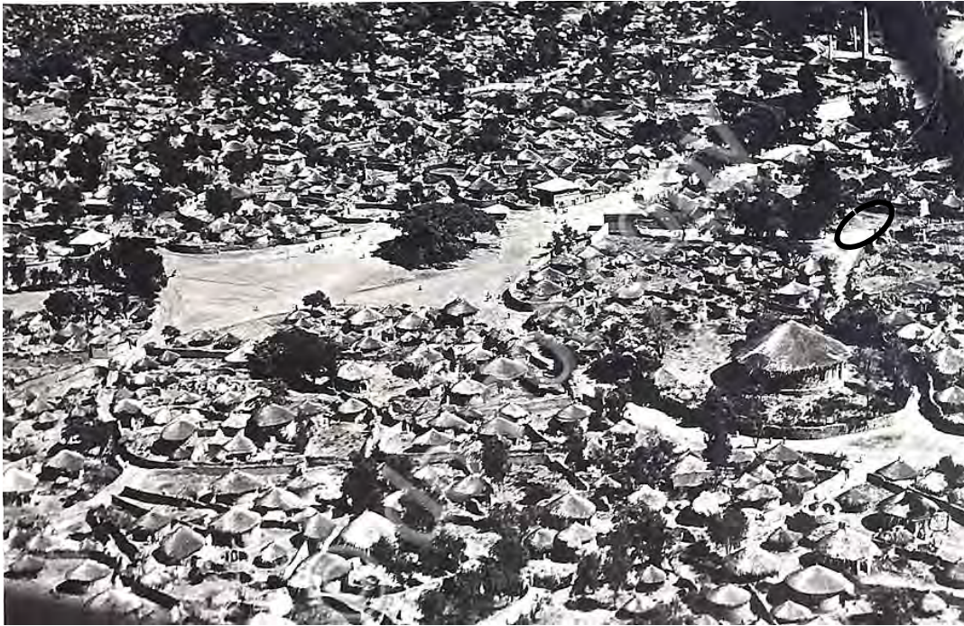
Fig. 5.46 Aerial view of the thrones site (in circle, right center) in the 1930s. The surrounding area of the sites was completely a built up area (Photo: available at: http://www.ebay.it/itm/Axum-Veduta-Aerea-Aerial-View-1935-36-Fotografia-Originale-Original/190826514657?pt=Fotografie_e_Stampe&hash=item2c6e2588e1 ).
