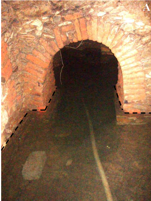
Fig. 6.1 The tomb of Brick Arch: (A) water filled up to the level indicated with broken lines. A plastic tube visible in the water was used to drain out the water. (B) View from upper stairs towards the interior; here a wet area can be seen when rainwater entered through the entrance and leaked through the side wall (upper right corner). A plastic tube used to drain out the water can be seen on the stairs (photo: Hiluf Berhe, 18/8/2008).
