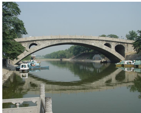
Figure 1.2: The Anji bridge, China.
